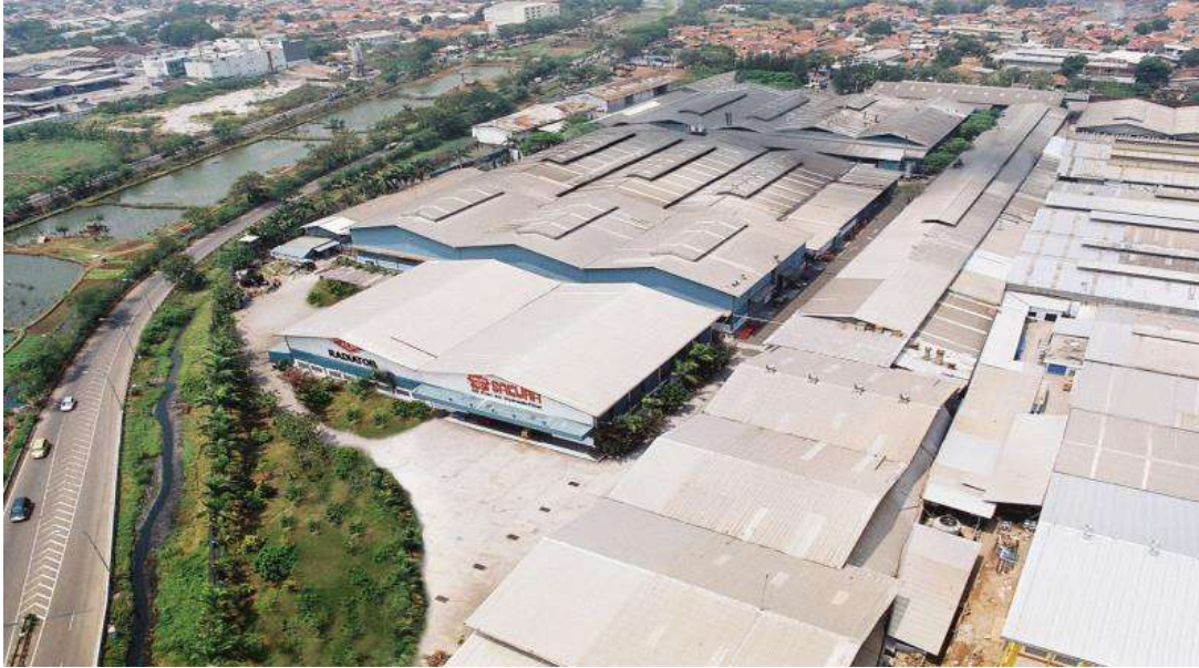
Kapuk Plant (Radiator Facilities)
